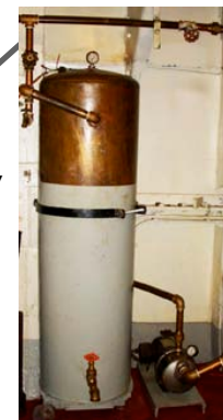
Domestic water system—copper tank made Jersey City, 1946
